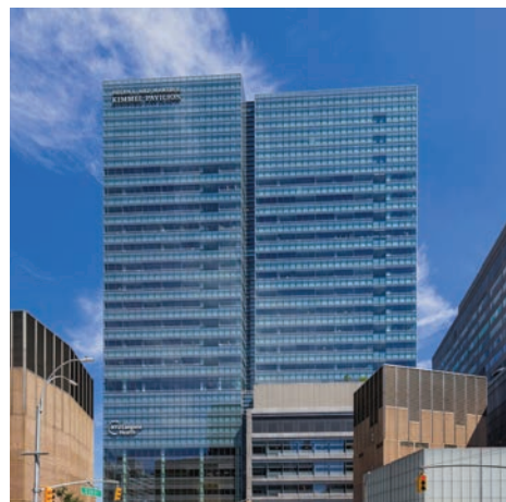
Kimmel Pavilion 900,000 ft 2 acute care adult & pediatric hospital LEED Platinum certified in 2019
